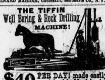
with this Machine! The most perfect in the world. Bores from 12 to 44 inches in diameter. It does he work of a dozen mea. The horse dozen to travel around the well. Auger is raised and lowered instantly. Successful where all others full. No labor for man. Send for our 60 PAGE BOOK, FREE.
