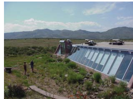
fig. 10p: Example of passive solar heating and proper building orientation, as implemented with the sustainability center (Ramsey, M)
