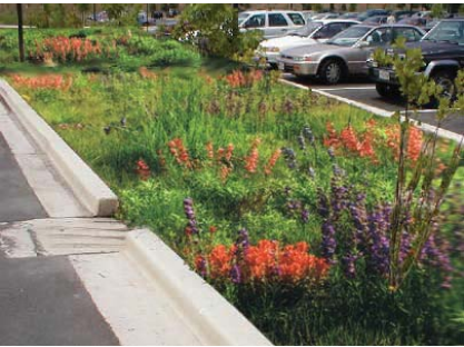
fig. 4i: This photoshop rendering shows the incorporation of native planting within a curb bioswale that will comprise the highway 54 boulevard. Stormwater enters the bioswale through the curb cut.
