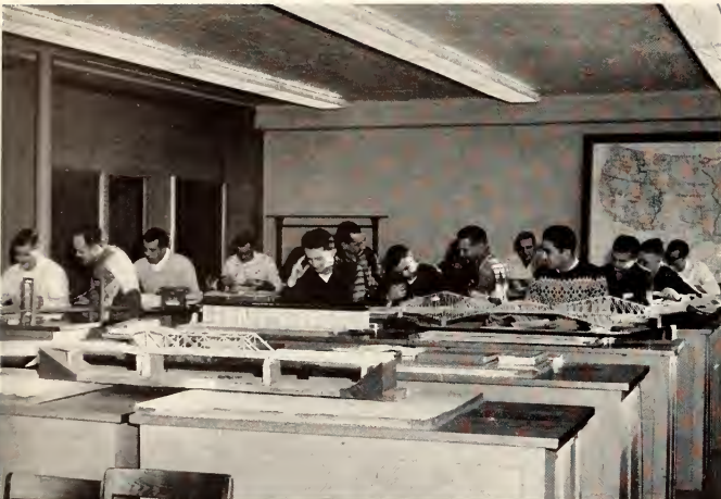
Constructing a bridge is a problem of vast complexity, even under model conditions, as these students are discovering.
