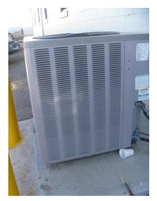
Figure B.17 Outdoor Air-Condensing Unit
