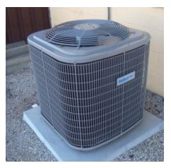
Figure B.31 Outdoor Air-Condensing Unit
