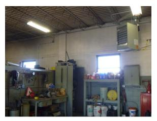
Figure B.21 Unit Heater in Storage Bays
