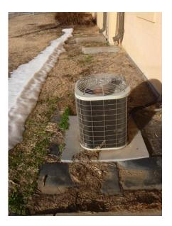
Figure B.42 Outdoor Air-Condensing Unit
