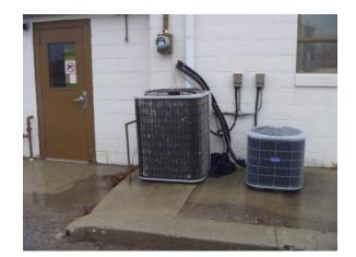
Figure B.9 Outdoor Air-Condensing Unit
