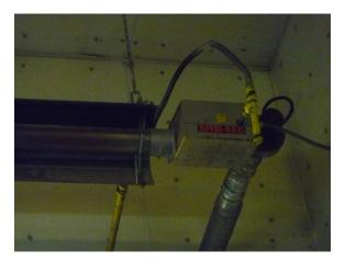
Figure B.41 Radiant Heater in Washbay
