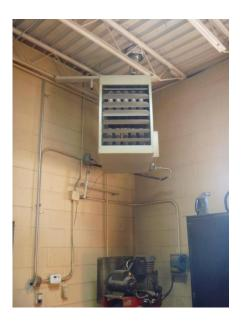
Figure B.38 Unit Heater in Garage Bays
