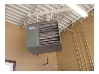
Figure B.36 Unit Heater in Garage Bays
