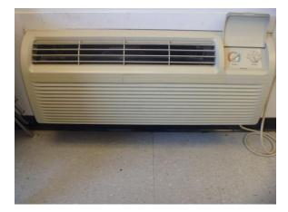
Figure B.27 Packaged Terminal Air Conditioner
