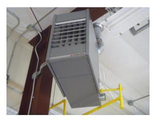
Figure B.25 Unit Heater in Garage Bays
