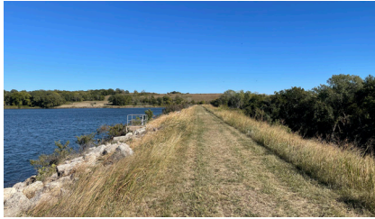
Figure 3.13. View of dam looking towards the site.
