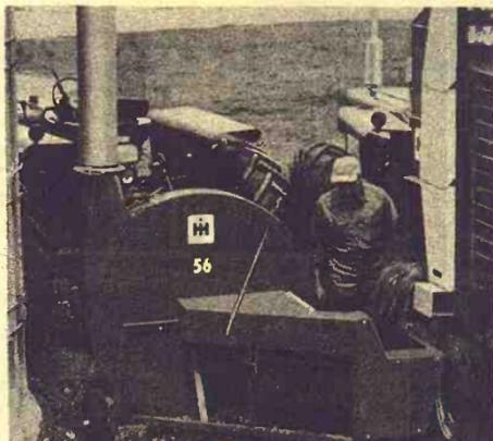
**International 56 blower.** Handles 100 tons of corn silage or 70 tons of haylage an hour, blows it 100 feet and higher. An exclusive 45° feeding system makes this huge capacity possible. It augers the crop in a near straight line flow to the big 56-inch diameter rotor. The direct-drive PTO takes 20 percent less horsepower than conventional blowers.
