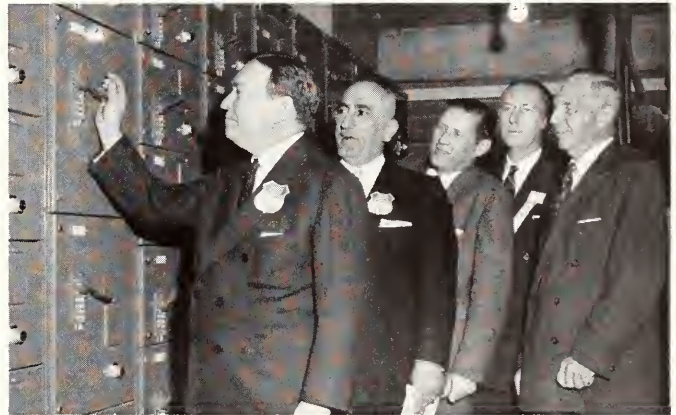
With a push of a lever , Benjamin Fairless, national industrial leader, sets K-State's new pilot feed mill into operation.
