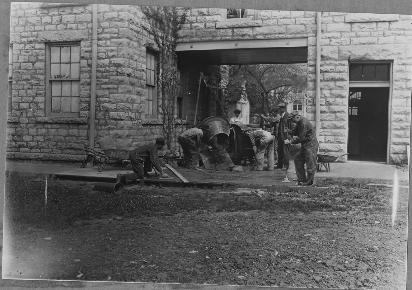
CONCRETE CONSTRUCTION CLASS, MAKING SIDEWALK IN SHOP COURT.
