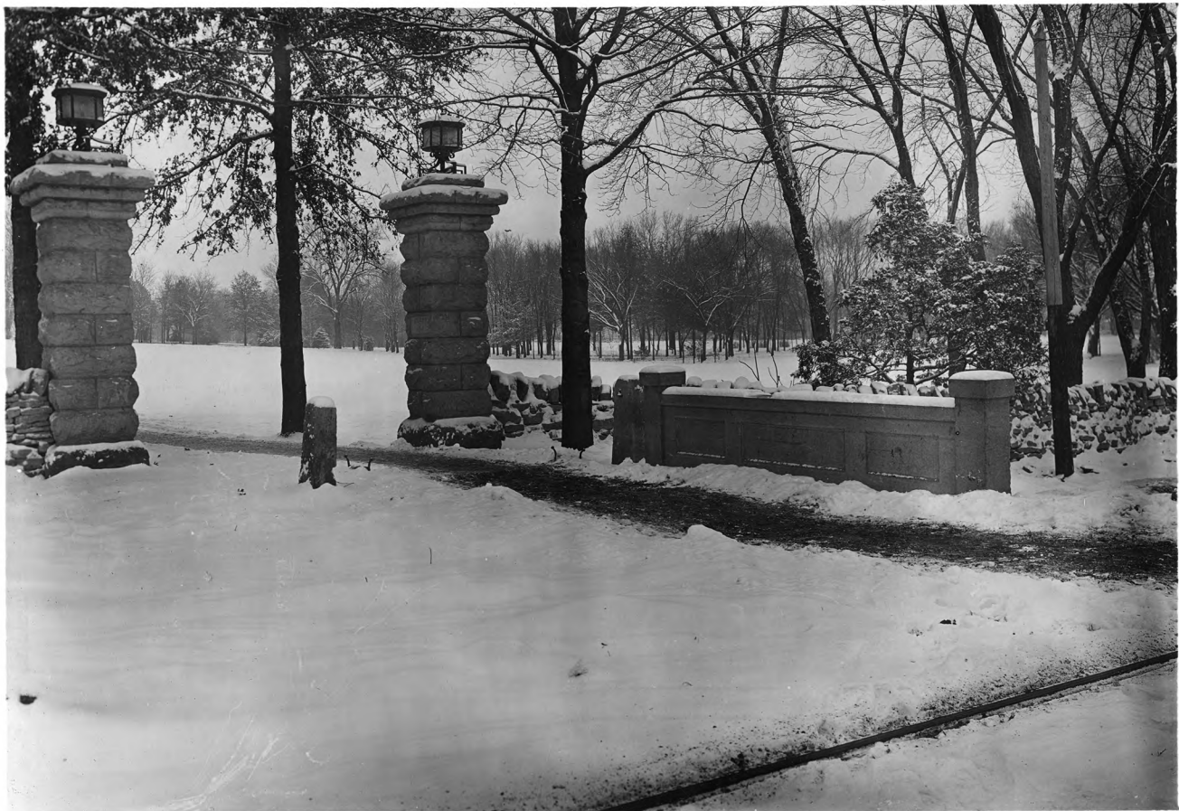
SOUTH GATE POST AND RAILING
