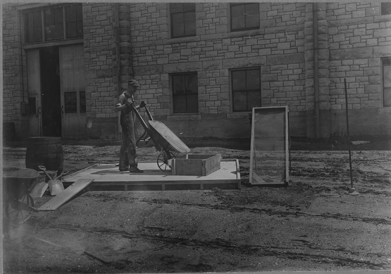
PREPARING TO MIX CONCRETE
