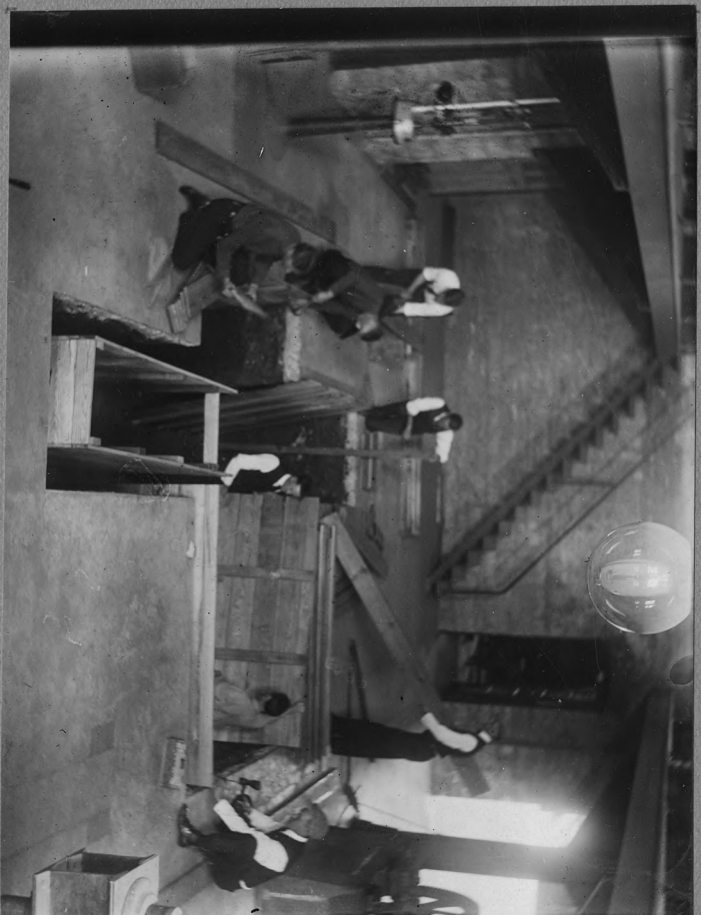
BUILDING FORMS OF OLSEN TESTING MACHINE
