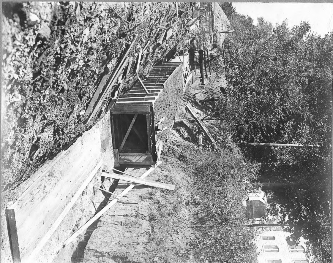
CONCRETE STORM SEWER
