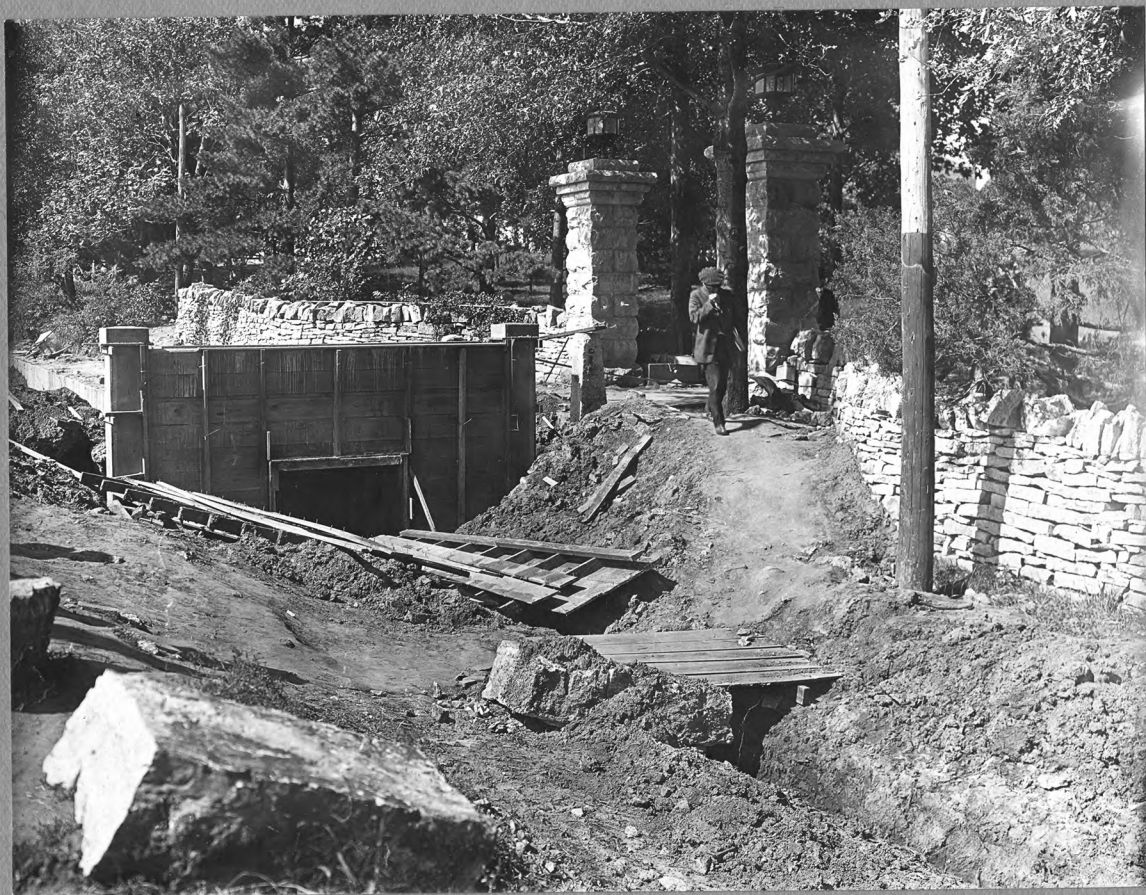
RAILING WITH FORMS AT SOUTH GATE
