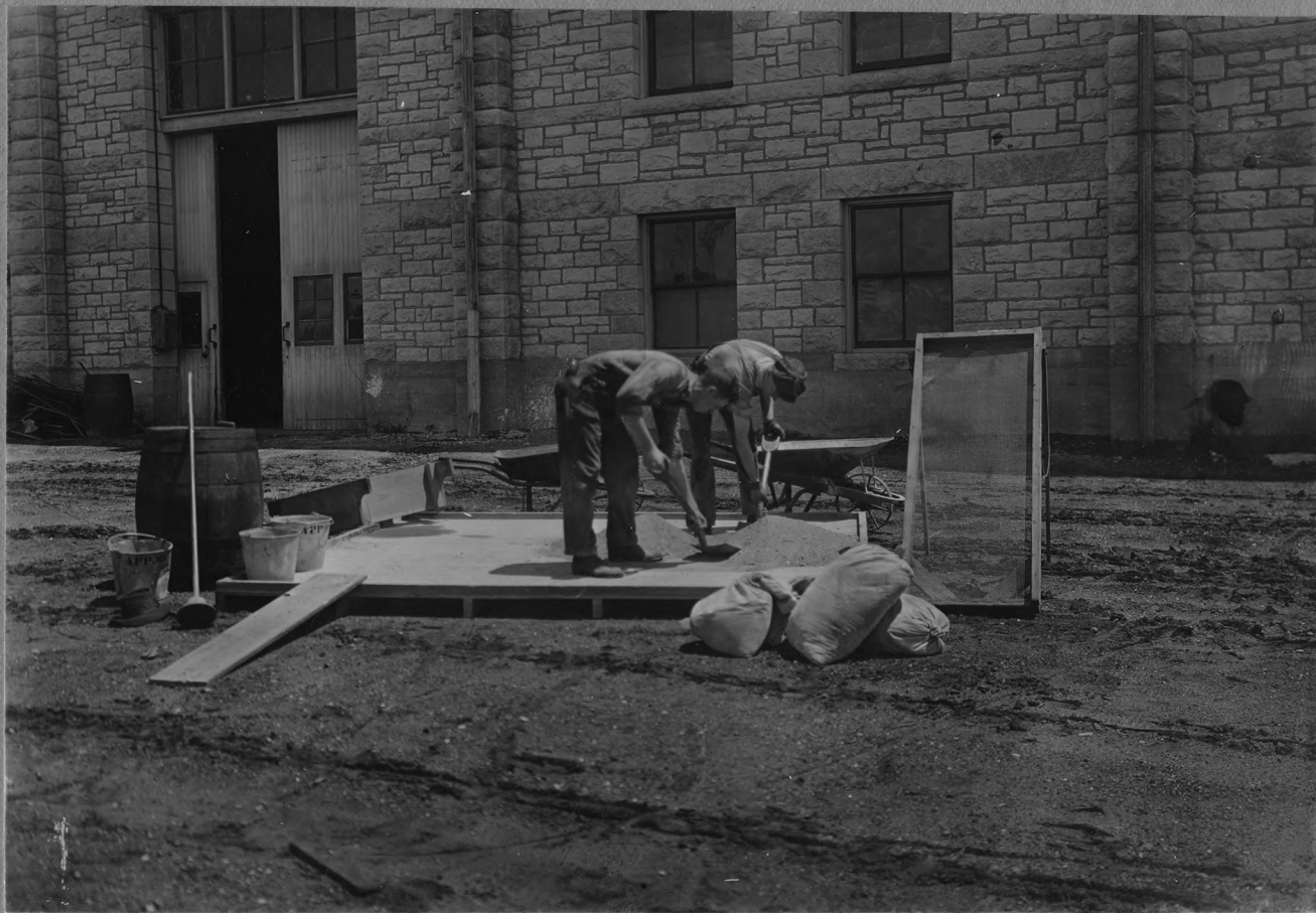
MIXING CONCRETE
