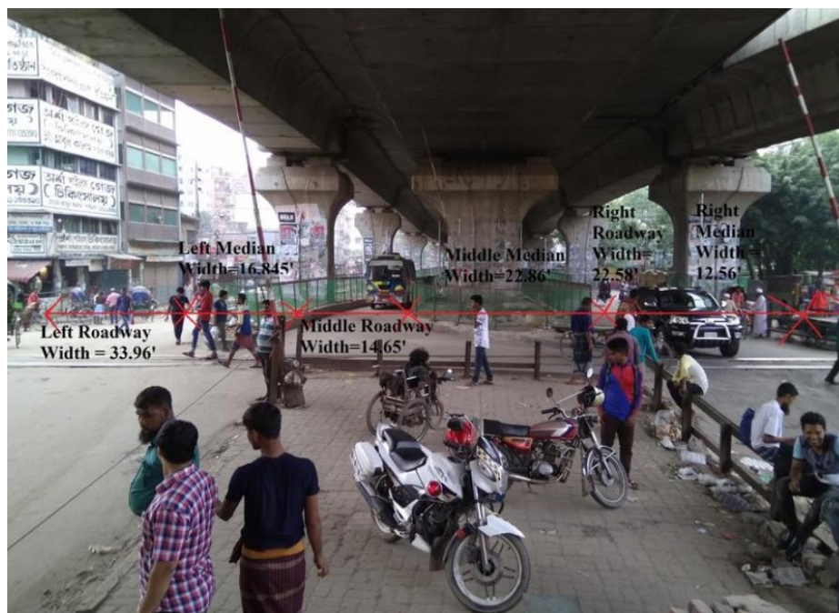
Figure 5.1: Existing rights of way reduction of “A H M Kamruzzaman Sarani” street by Mayor Mohammed Hanif Flyover
