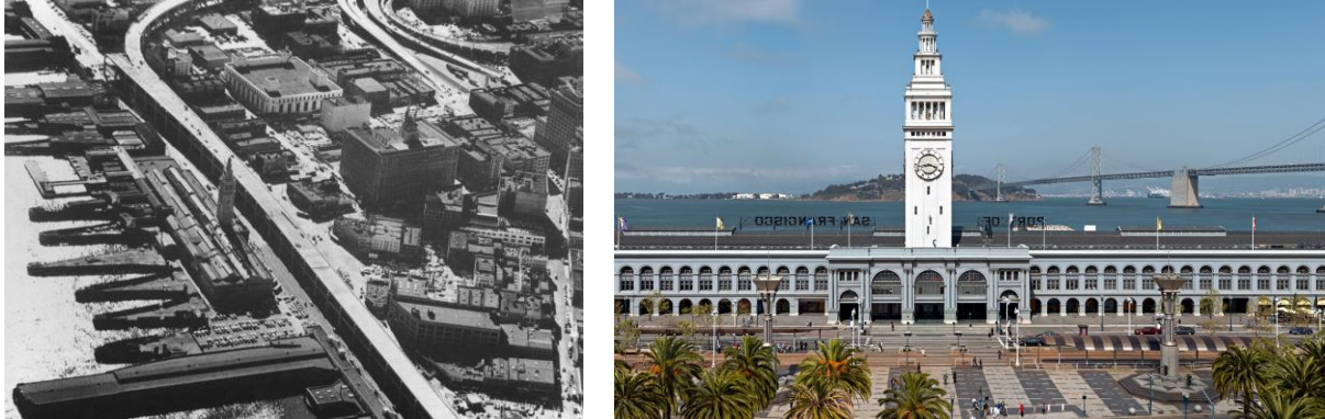
Figure 2.3: Embarcadero Freeway and Ferry Building, in 1960 (left); Renovated Ferry Building and boulevard today (right)
