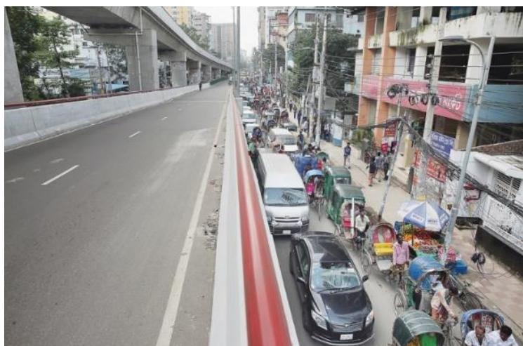
Figure 3.17: Traffic gridlocks still exists on streets while Moghbazar-Mouchak flyover remain unused
