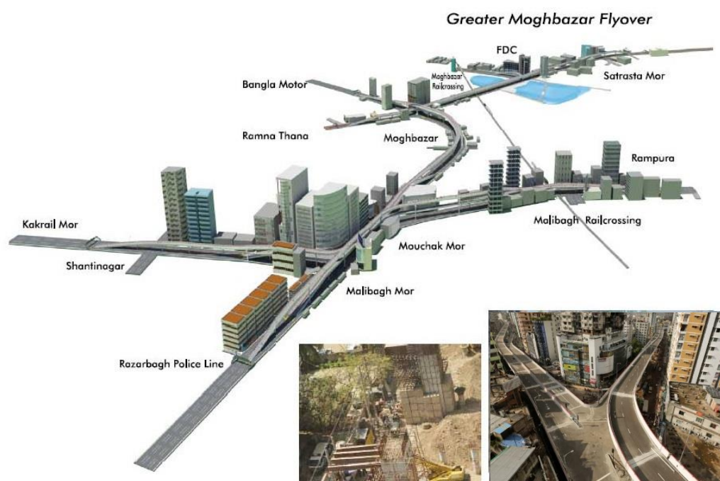
Figure 3.10: Moghbazar-Malibagh Flyover, completely opened in 2017
