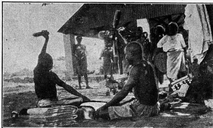
Ironing Cloth After Washing, or Dyeing; the Cloth is Folded Several Times and Then Pounded as Shown on Flat Rocks
