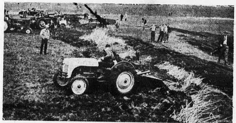
Machinery dealers used $150,000 worth of machinery to complete a one-day soil-conservation job on 3 Shawnee county farms, April 19. Here, some of the equipment is shown filling a ditch preparatory to putting in a seeded waterway.
