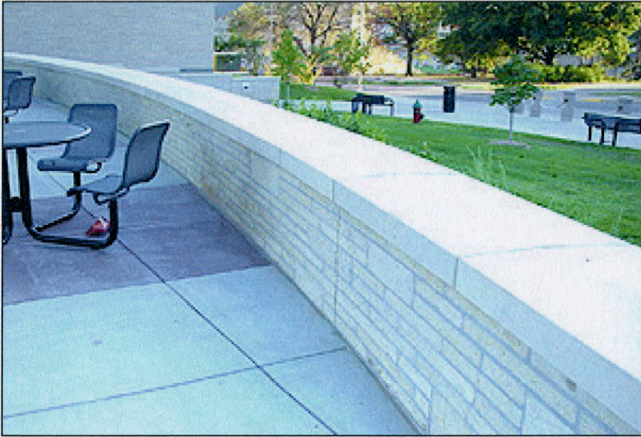
Figure 5.15: The retaining wall on the western side of the outdoor eating area.
