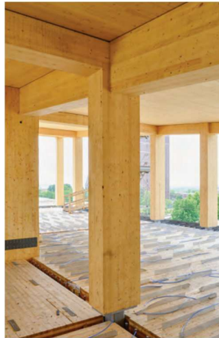
Figure 8 Olvern Design Building Before Concrete
