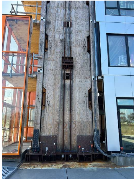
Figure 8. Rocking Wall (Post, 2023)
