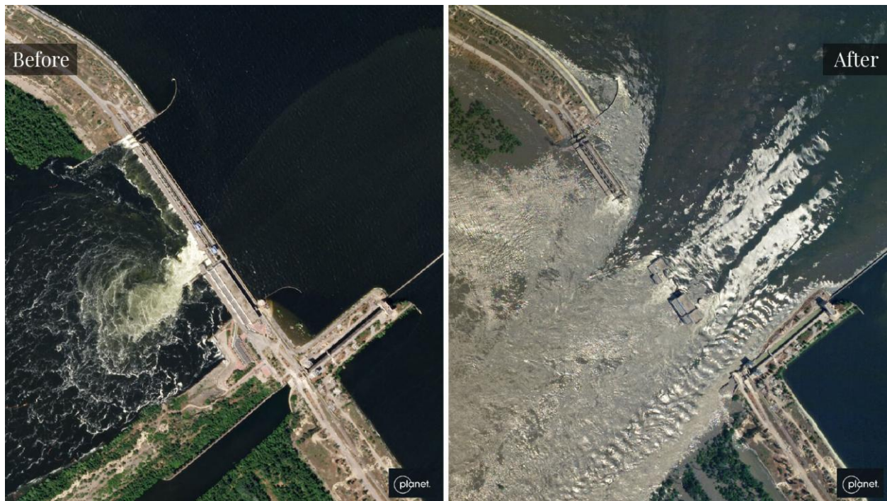
Figure 2-6: Before and after satellite images of Nova Kakhovka dam - This figure shows pre- and post-event satellite imagery of the Nova Kakhovka Dam, highlighting structural damage and downstream flooding following its destruction ( Satellite Images Show Ukraine's Kakhovka Dam after Destruction | Russia-Ukraine War News | Al Jazeera , n.d.). It is analytically important because it illustrates the large-scale environmental and hydrological disruption caused by conflict-related infrastructure damage.
