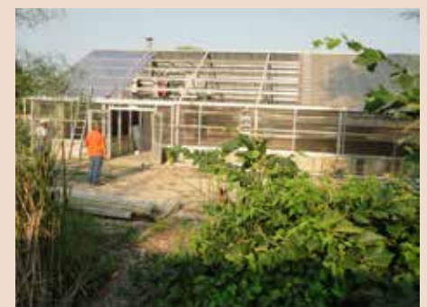
Contract employees working on greenhouse renovations. The fiberglass to the left is new and to the right is the fiberglass from 1993.
