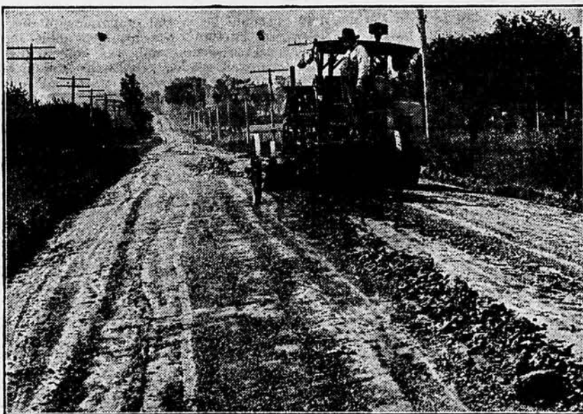
SHAWNEE COUNTY DIRT ROAD IN PROCESS OF CONSTRUCTION. — COMBINATION TRACTOR AND ROLLER PULLING GRADER
