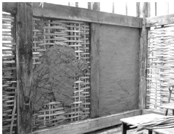
**FIG. 6 WATTLE AND DAUB CONSTRUCTION**
