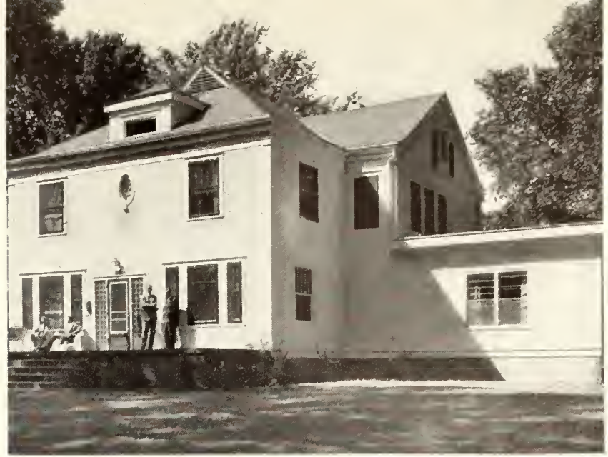
THETA XIS at 1614 Fairchild have done extensive remodeling and building on their present home.
