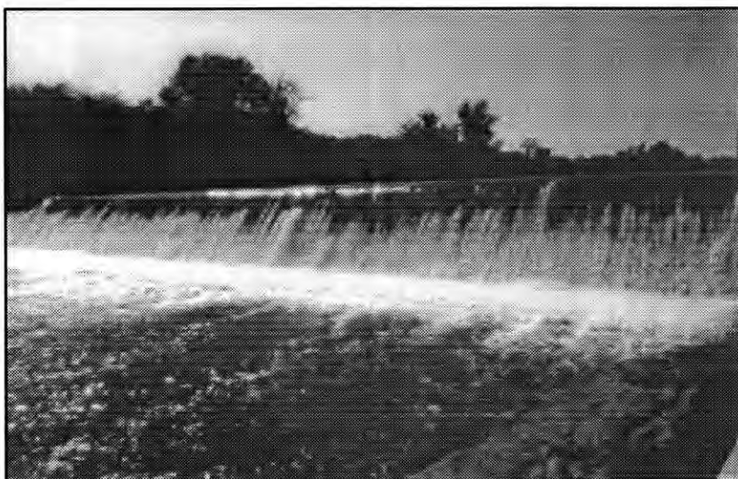
FIGURE 57. Rocky Ford Dam as seen looking west, has a 10 to 14 foot (3.0-4.8 m) drop in elevation. Elevation drop depends on backwater effects from the Kansas River. (Photo by: Author 1991)
