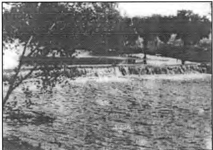
FIGURE 23. Purcell Dam, shown here in an 1870 photograph, was constructed in 1860. The dam was used to mill grain for ten years and then sat idle for 40 years before being developed to generate electricity (Photo courtesy of Riley County Historical Museum).
