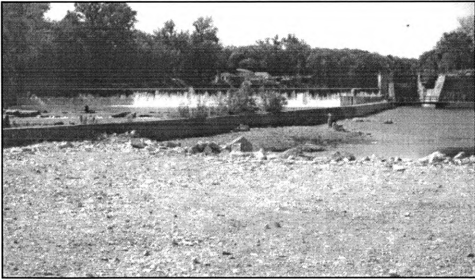
FIGURE 25. Rocky Ford Dam, photographed facing northwest, in May of 1992, is still a favorite spot for local anglers. The retaining wall was reconstructed in the summer of 1988 to improve angler access to the river. (Photo by: Author)
