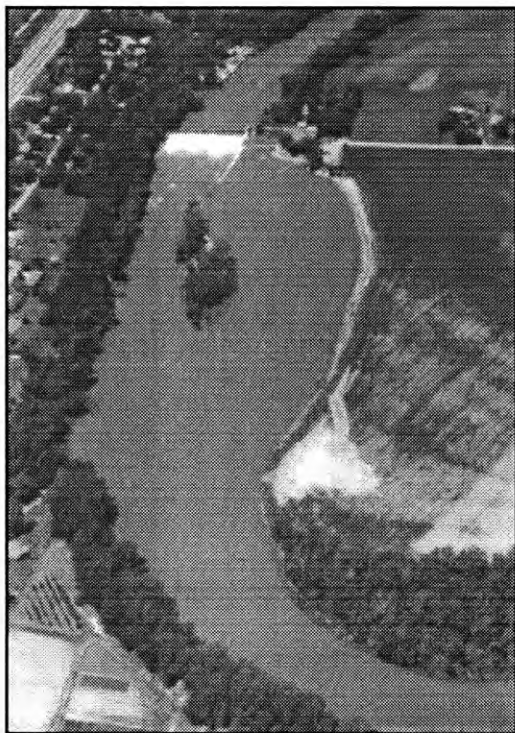
FIGURE 56. Rocky Ford Dam photographed from the southeast, located 1.4 miles (2.2 km) downstream from Tuttle Creek Reservoir. (Photo by: Author 1991)
