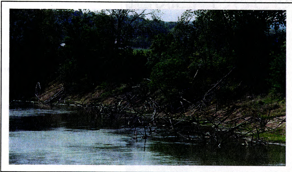
FIGURE 61. Rehfield jetties immediately upstream from the Casement Road Bridge, along the northern bank. Casement Road Bridge is 2.5 miles (4.0 km) downstream from Tuttle Creek Reservoir. (Photo by: Author 1991)
