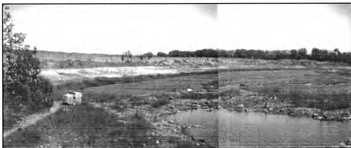
FIGURE 58. Below Rocky Ford Dam viewed from the west, bank erosion can be visually identified during periods of low discharge. (Photo by: Author 1991)
