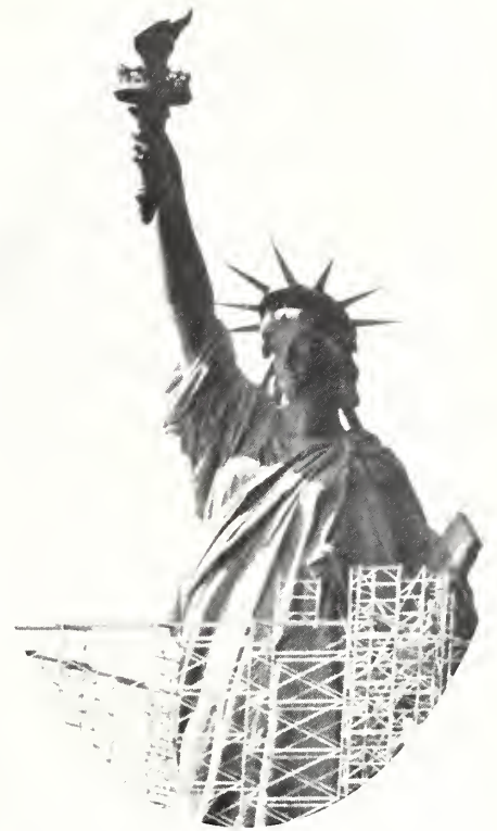
The Statue of Liberty celebrated her 98th birthday in 1984 and she began to show her age. The statue was worn from constant pummeling from wind, salt air and acid rain, and the iron ribbing supporting the copper covering was corroded. A two-year restoration began in July 1984. It included a new goldplated torch. (AP/Wide World Photos)
