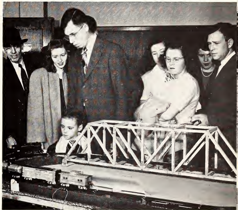
THE CIVIL ENGINEERING EXHIBIT also included a model bridge wired to show various stress points when crossed by a model train.
