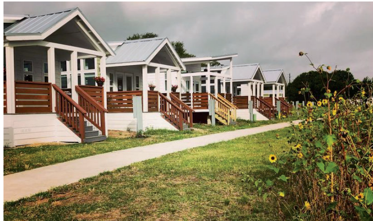
Figure 4.40 Village Farm: Architectural Character (Village Farm Austin 2021).
