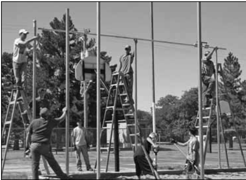
Grainfield volleyball court construction.
