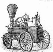
THE AMES THRESHING ENGINE. This make of Engine is used and recommended by nearly every manufacturer of Treshing Machines who does not make engines. They are the most complete "mounted" Engine now in the market. We furnish steam and water gauges, governor, whistle, etc., with the Engine. Send for illustrated pamphlet.
