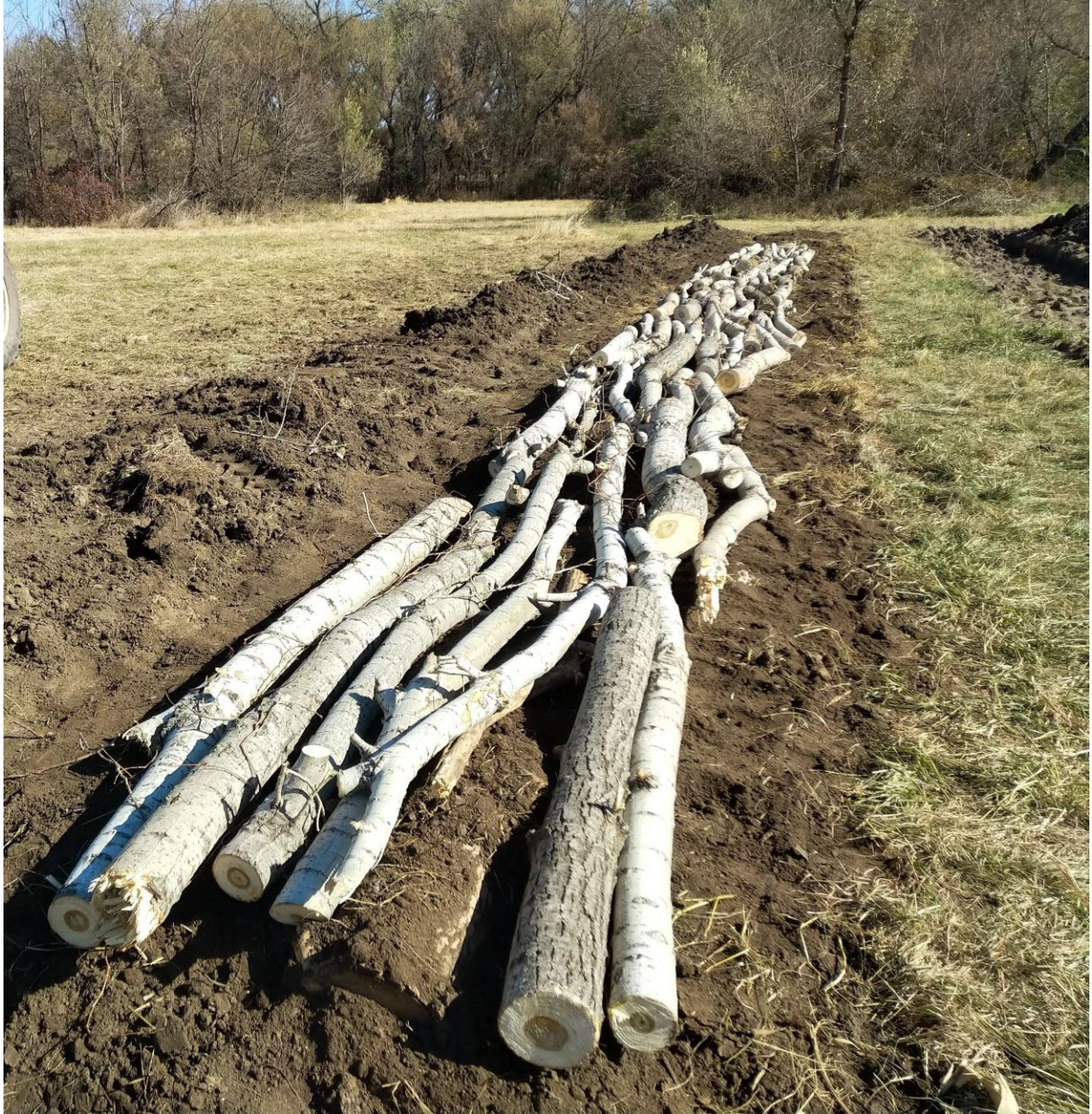
Figure 3. During the hügel bed construction process, the second layer of the hügel bed starts by adding slightly smaller wood on top of the tamped and raked soil and compost mixture of the first layer at Kansas State University's Willow Lake Student Farm.
