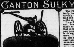
The Plow at all times will run perfectly level. The horses are attached directly to the end of the beam; the land and depth are guaged by a clevis at the end of the beam.
