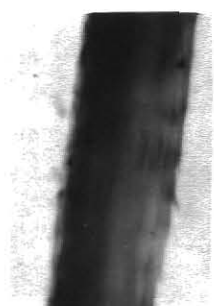
FIGURE 5 LOOSE AND ROUGH SCALES
