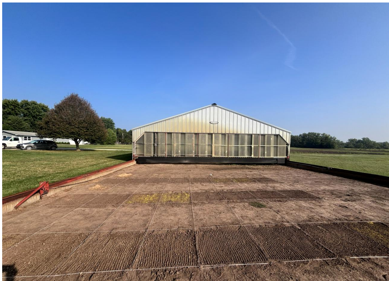
Figure D.1. Automated rainout shelter used for field experiments at Rocky Ford.
