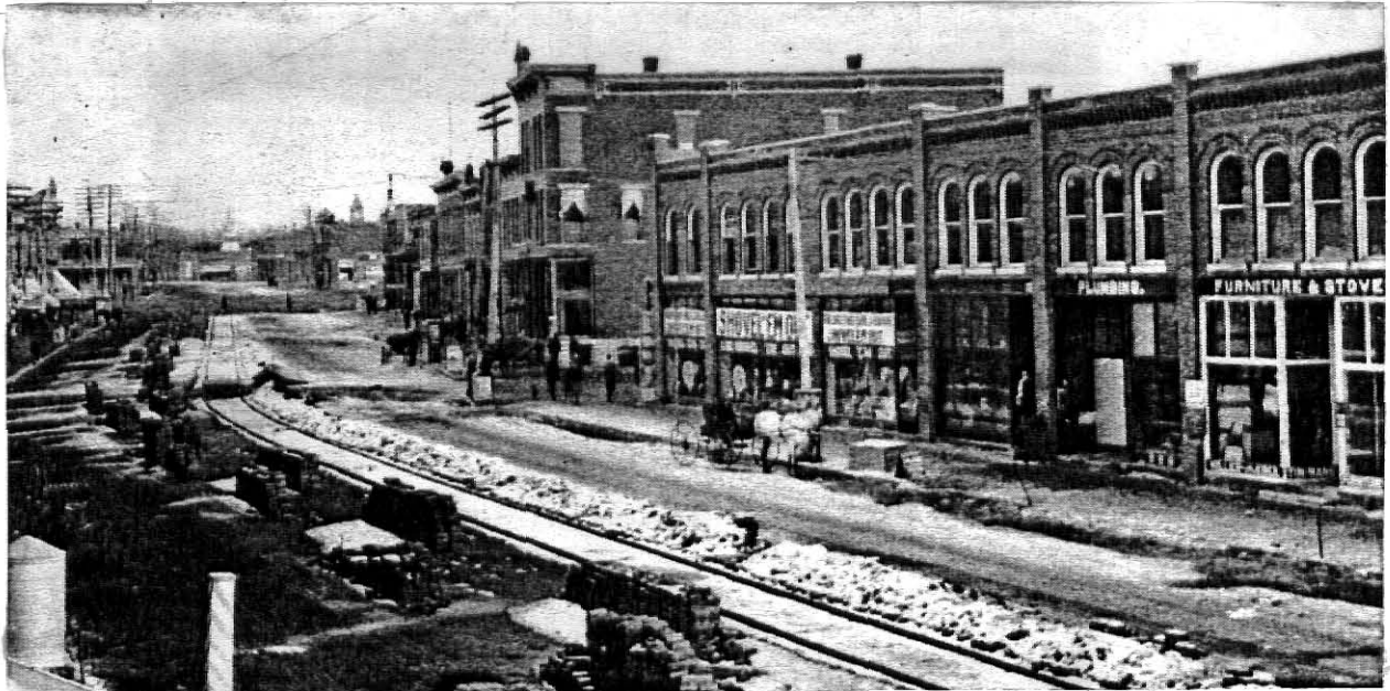
Construction of Union Electric Interurban Figure 15
