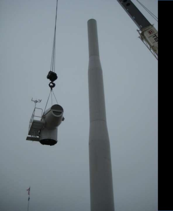
Picking the nacelle up to install it on the tower.
