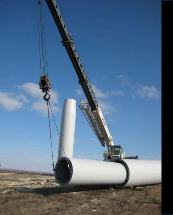
Un-nesting the upper tower section from the mid-section. The lower section has been installed behind the crane.
