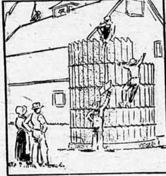
No. 10 They are putting up the silo. It is easier and quicker than Bill even expected. The Lock-Joint Cement Staves fit—one into the other and form one continuous, yet pliable wall. Mrs. Williams really enjoys talking with the man sent to put up the silo.
