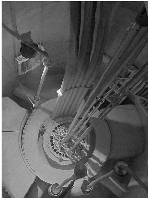
Figure 6-15 The Triga Mk II nuclear reactor core is shown. The control and fuel rods are labels along with the IRIS port numbers 1 through 6.
