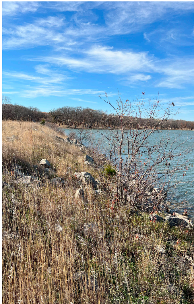
The dam is armored with large rocks and established tallgrasses. The lake bottom drops off quickly from the face of the dam to deeper water.
