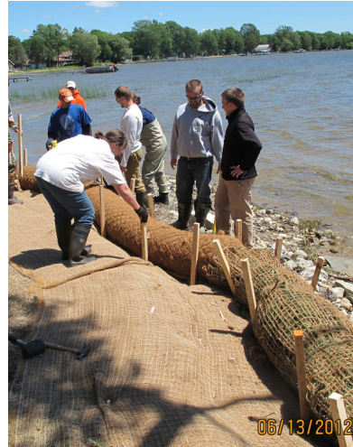
Fiber rolls and burlap netting are installed to initiate shoreline stabilization.
