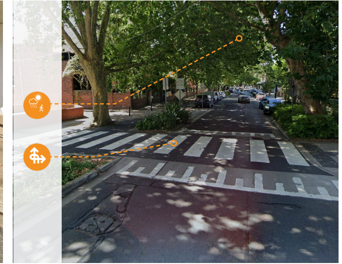
Figure 4.14: Bourke Street Raised Intersections | Image Credit: Google Earth
