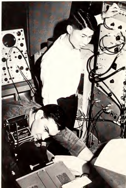
New equipment for the electrical engineering department includes this machine which takes pictures through use of radar.
