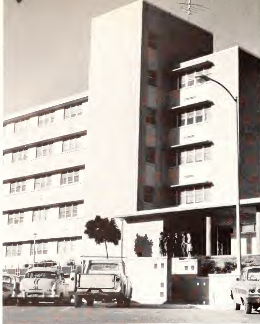
West women awaken mornings to construction sounds from work on one unfinished hall in a four-dormitory complex.
