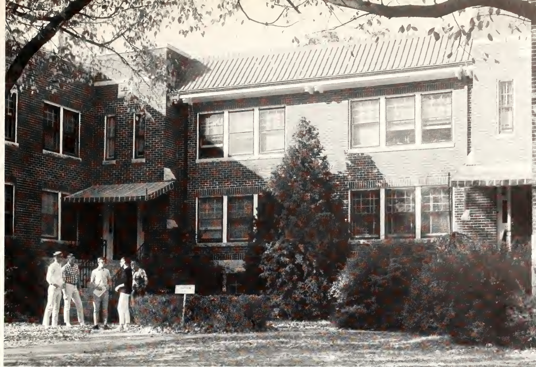
Formerly an all women's dormitory, Waltheim hall, 1436 Laramie, now houses both men and women. Although it is a Uni-
