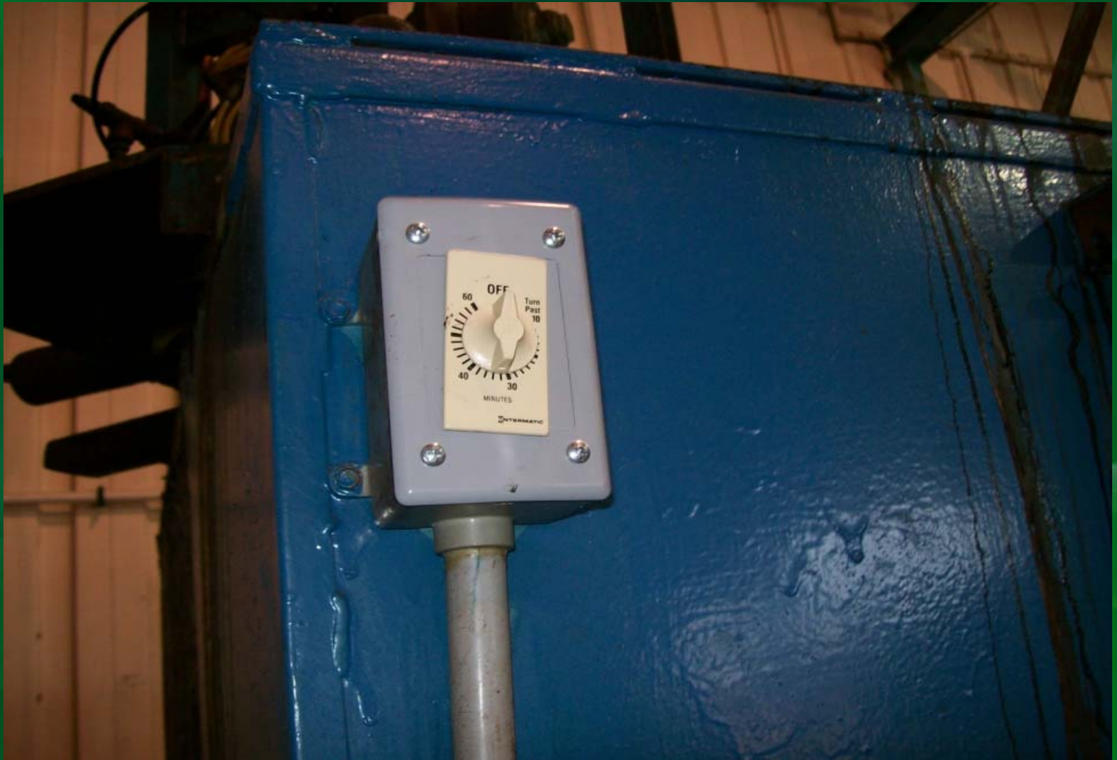
Fig.: Installation of a timer
