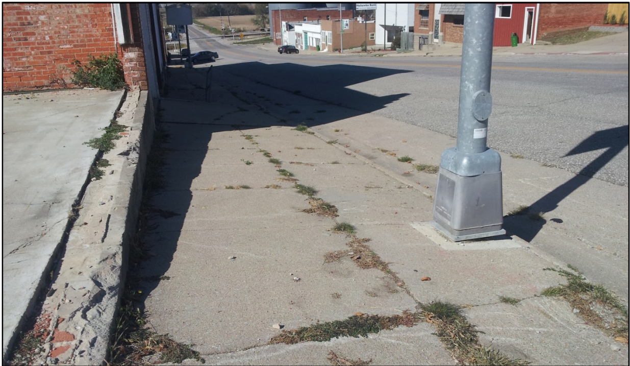
Figure 7.3: Sloped and dilapidated sidewalk down Main Street in Union, Nebraska.
