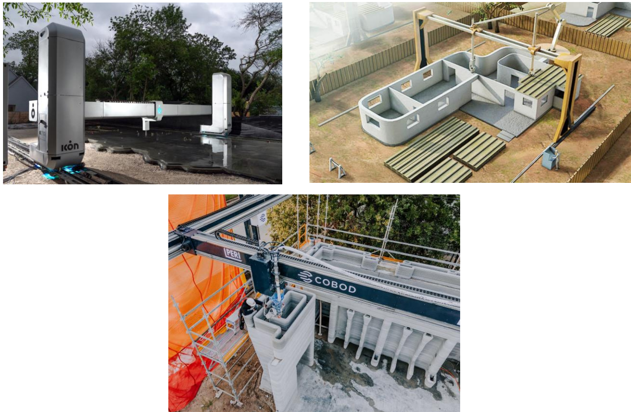
Figure 1: Examples 3D concrete printer setups (Molitch-Hou, 2021), (Link, 2015), (HANNAH, 2022)
