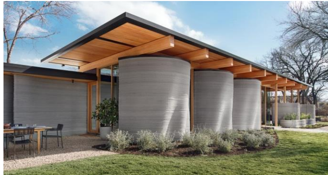
Figure 2: Examples of complex geometry made possible through 3D concrete printing
