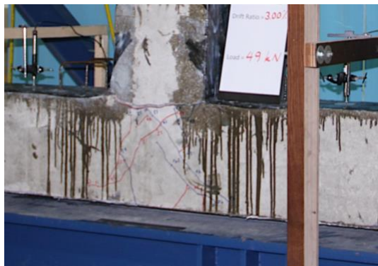
Figure 2.2. A Closer View on The Column Critical Section Where Failure of The Four Specimens Occurred (Saqan et al. 2020).
