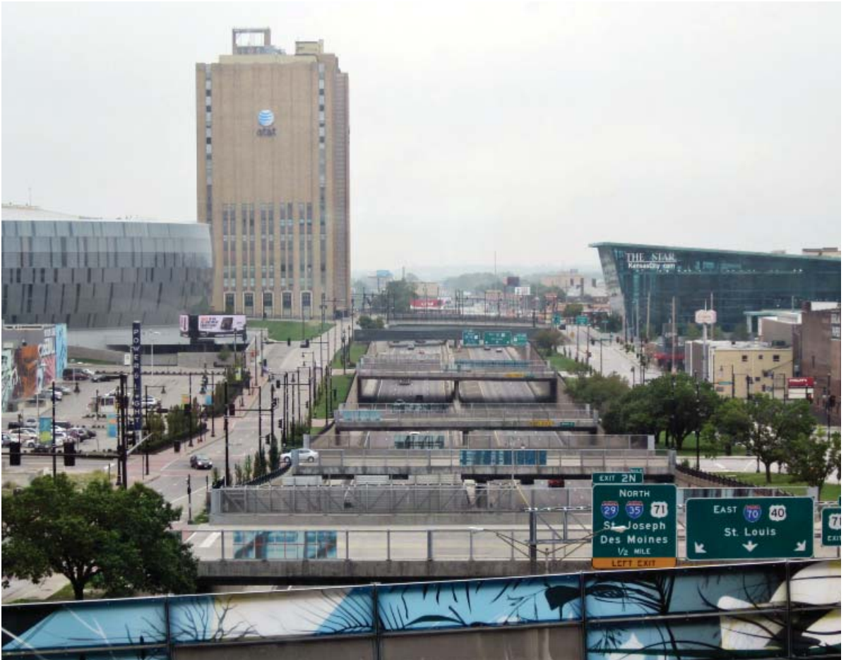
Figure 4.09: Corridor View East from Bartle Hall Convention Center
