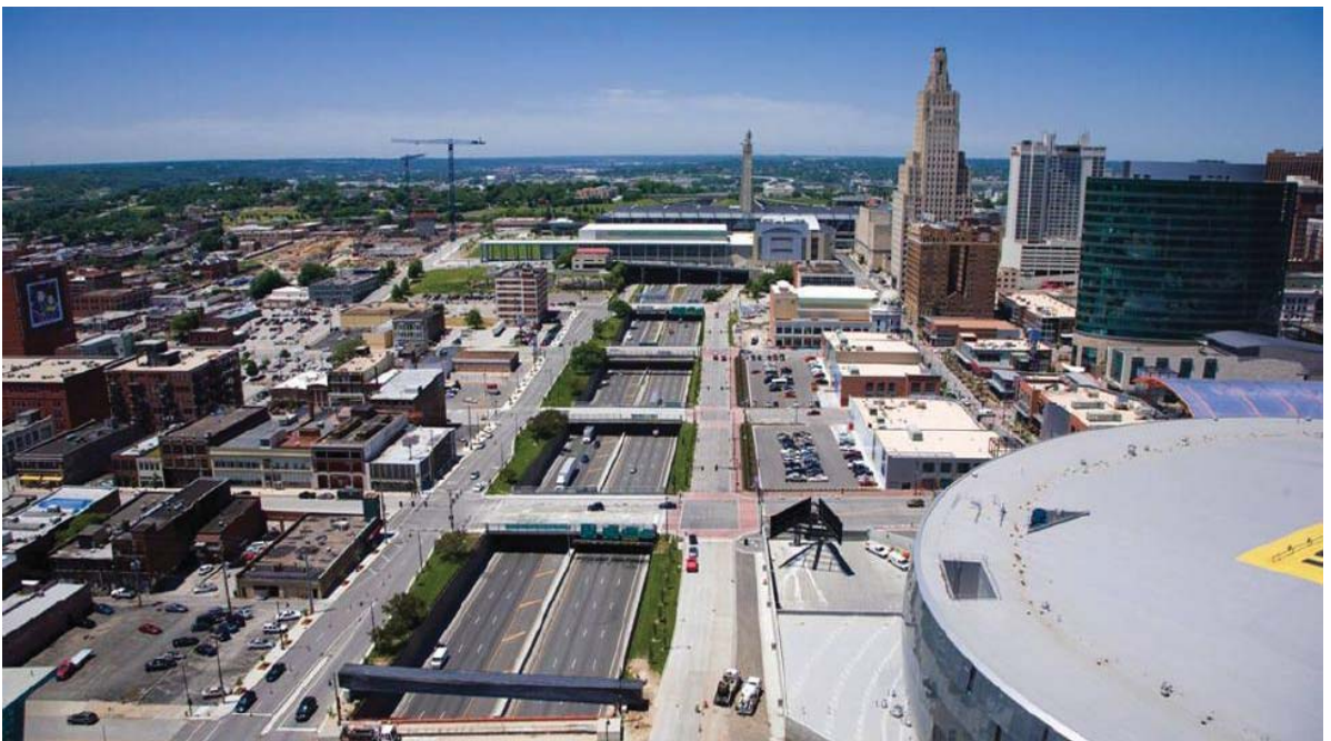
Figure 4.10: Corridor View West
