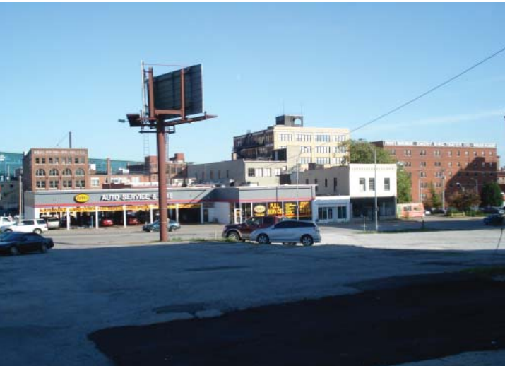
Figure 2.09: Surface Parking Lot
