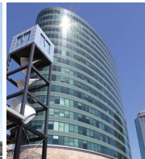
Figure 2.13: H&R Block Headquarters
