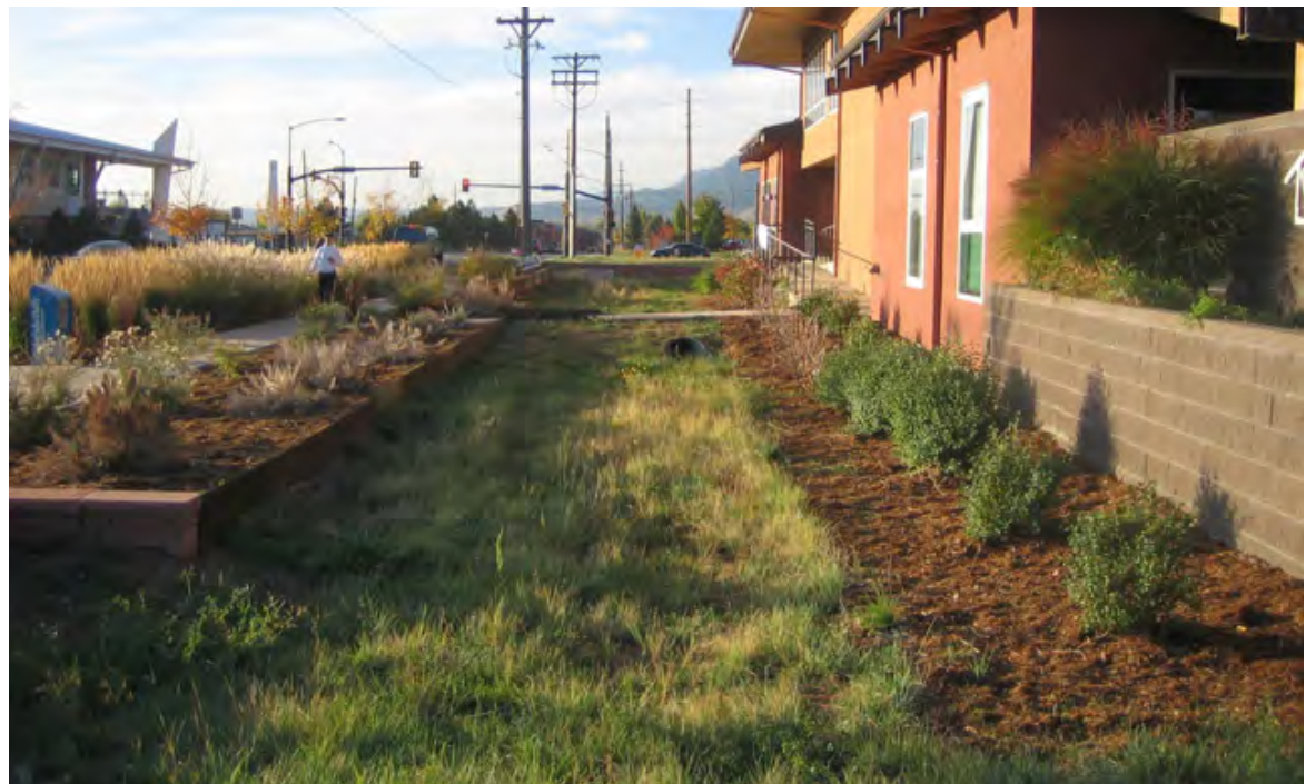
Figure 7.34 Bio-Swale in Boulder, Colorado ( www.dkahn.com )
