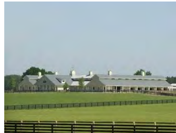
Figure 2.11 Oaks Exterior View (www.eqsv.com)
