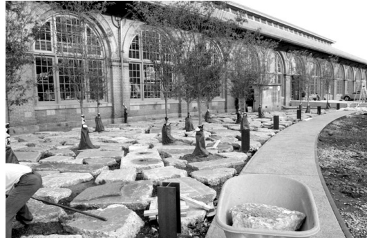
Figure 4.33. Urban Outfitter Corporate Campus, Philadelphia Navy Yard . The plaza by DIRT Studio is composed of recycled concrete pavement. Once again existing sidewalks can be recycled and incorporated into the design. In the perspective to the right recycled concrete pavement is used to create a space within a space at the Maplewood MetroLink station ( http://www.arch.virginia.edu/lunch/print/territory/sustaining.html ).
