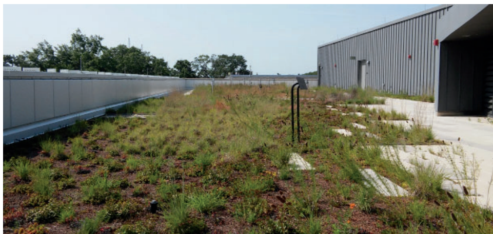
Figure 10: Rooftops Designed or Used for the Support of Vegetation Growth, Recreation, Aesthetics, and Noise Reduction. (Skabelund, 2021)
