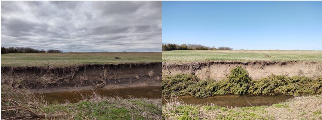
Figure 2. Second redcedar revetment installation during early spring with low water levels (before/after)
