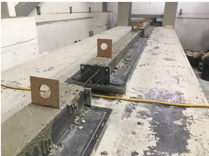
c) All concrete placed
