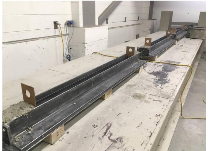
b) Concrete with fiber placed
