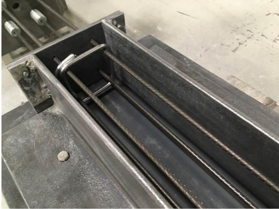
Figure 83. Stirrups preparation and set up
