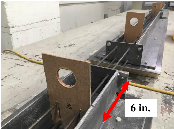
a) Framework ready for concrete
