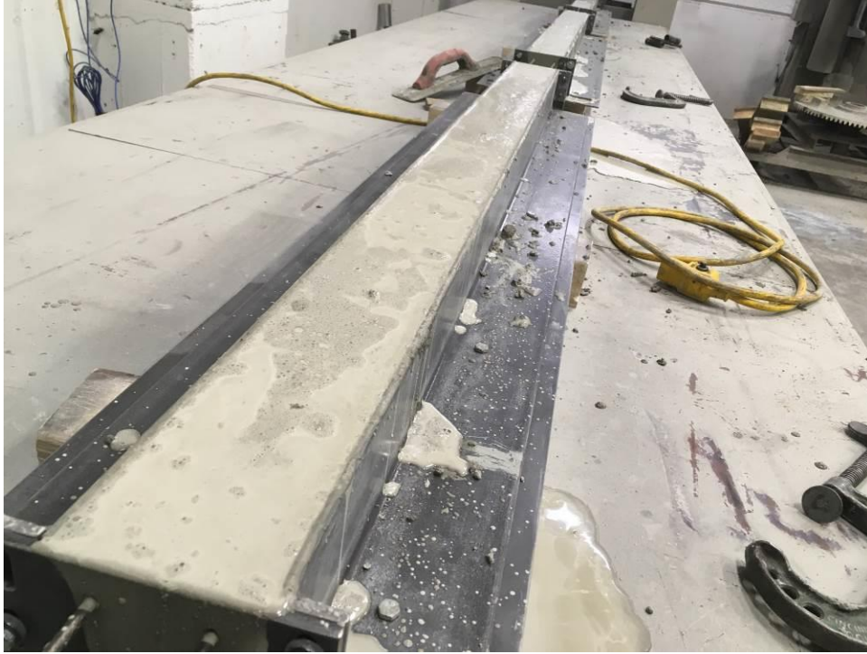
Figure 65. Prims made of segregated mix after placement and consolidation (B161)
