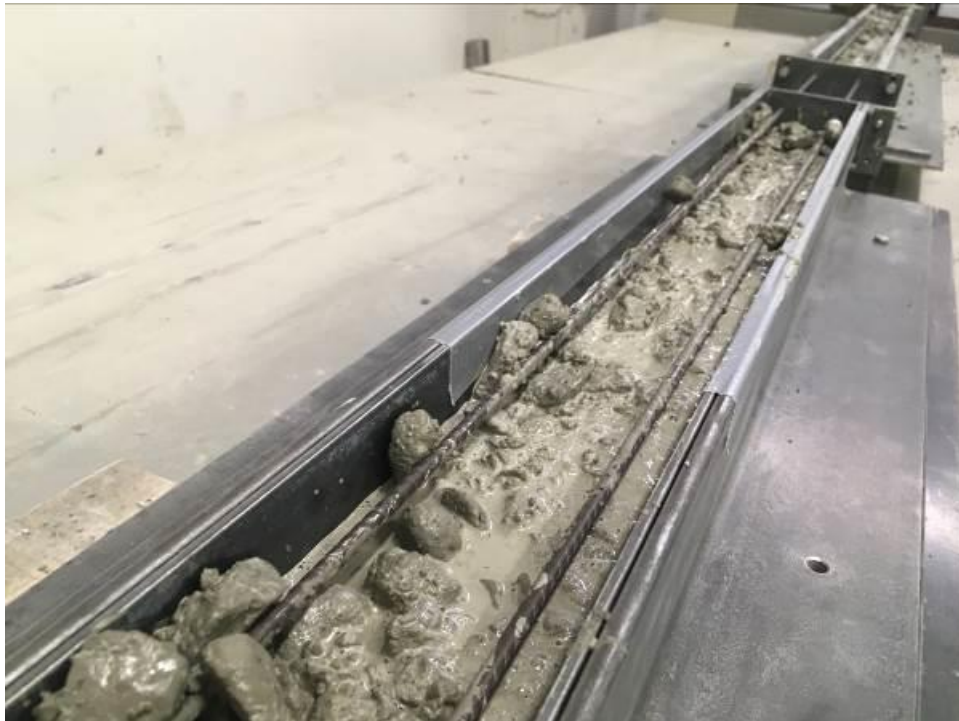
Figure 64. Segregation of Mix B161 during casting
