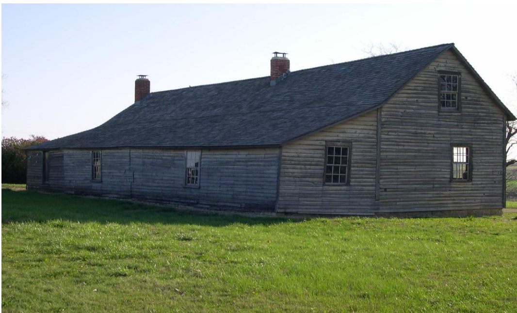
Figure 6: The Hollenberg cabin as it appears today, looking to the northeast. The west-end addition is highlighted in this photo. Source: Ashley Rhodes, 2012.
