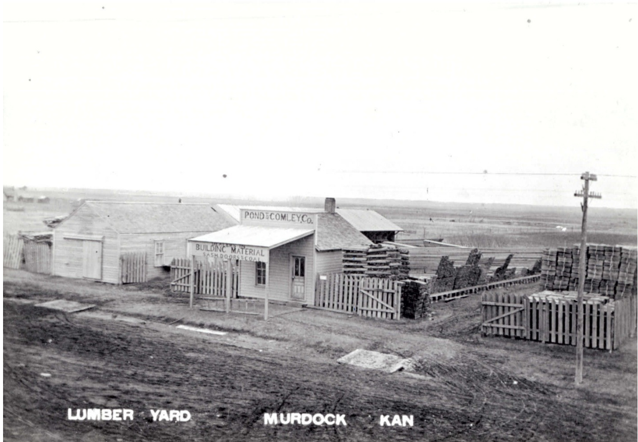
Figure 10. Photograph of the lumberyard in Murdock, KS ca. 1912. Photo courtesy of Kingman County Historical Museum.
