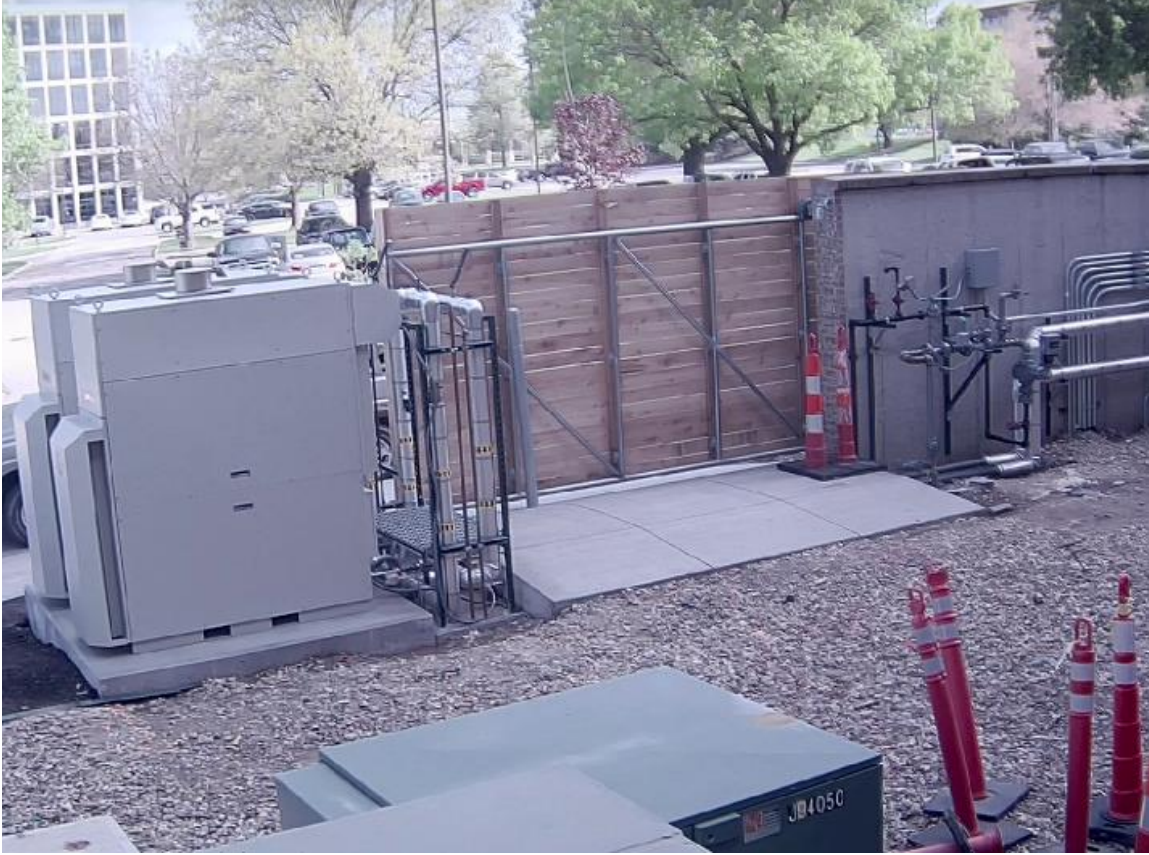
Figure B.17: Black & Veatch world headquarters microturbines.
