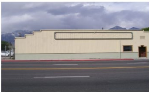
Mairs Market Building before construction
